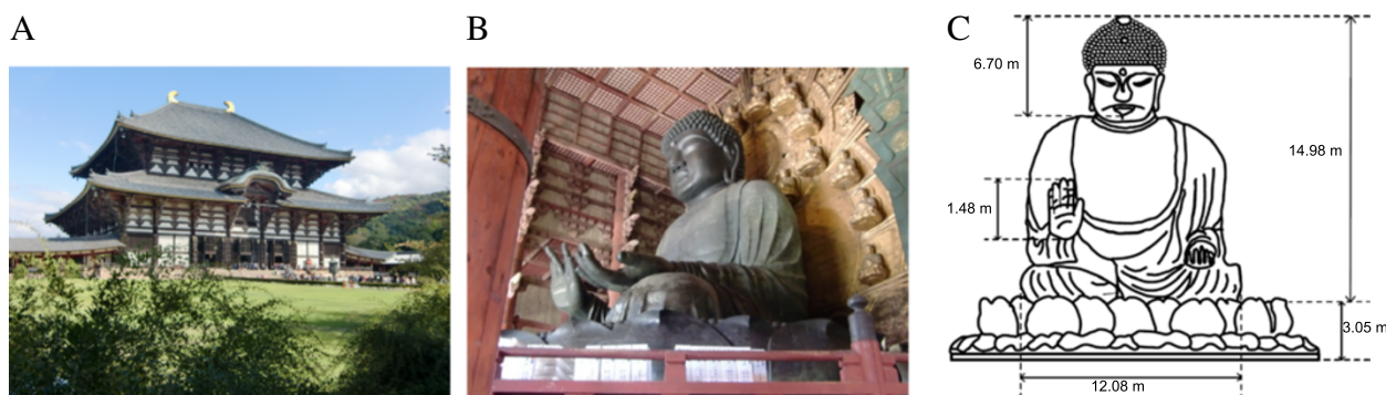
Figure 2 Photographs and schematic representation of the Nara Daibutsu. (A) Current Great Buddha Hall (Daibutsuden), which is 57.5 m wide, 50.5 m deep, and 49.1 m tall. It was rebuilt in 1691 A.D. due to fire. The original hall was even larger and had a width of 86 m. (B, C) Great Buddha. Processes involved in the production of the Buddha were as follows: More than 2 million people were reportedly involved in this project, even though the total population of Japan was 5 million at that time (Kito 2000).
